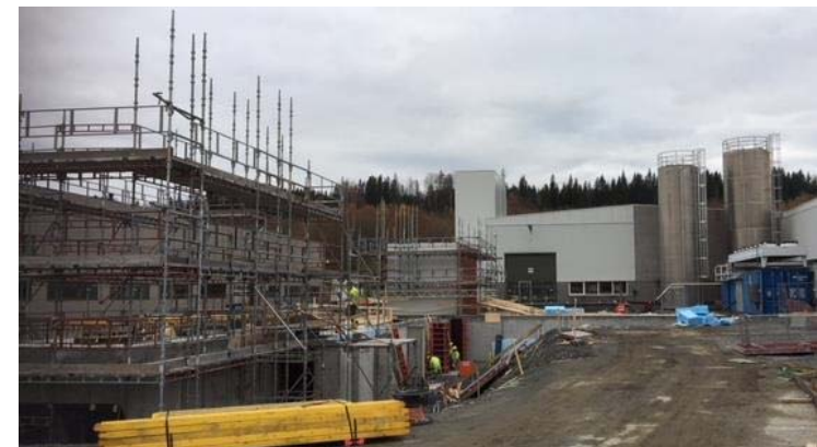
Construction work at Raufoss, October 2017
