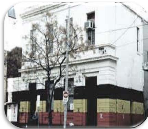
VAHS's second building at 136 Gertrude Street into which the Service moved in 1979.
