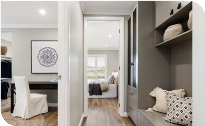
2340mm high passage doors to ground floor & 2040mm to first floor
