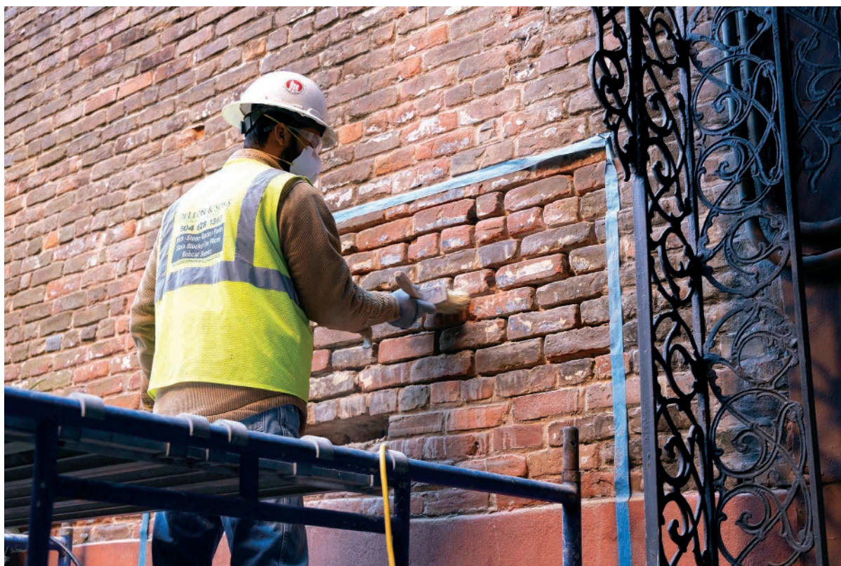
A. Brick courtyard walls get a preservation-minded touch-up by a contractor from DeLeon and Sons.
