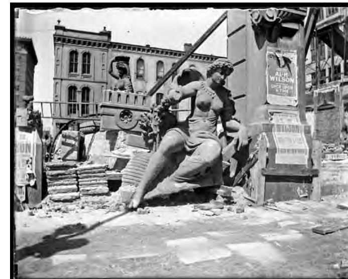
The demolition of the New Orleans Cotton Exchange, 1919 (2003.0182.166)
