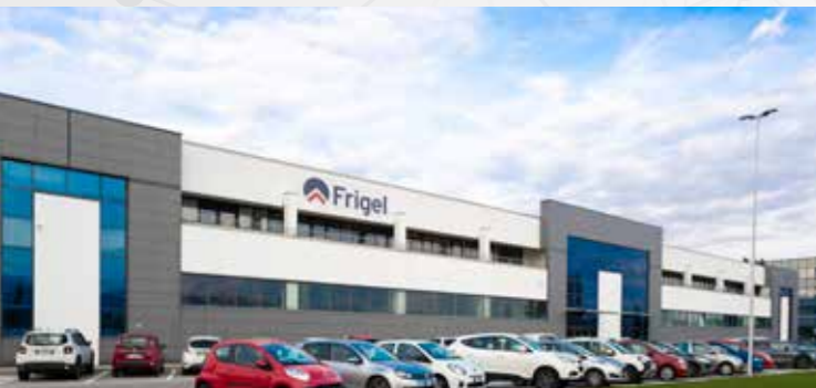
FRIGEL Firenze Headquarter Manufacturing, Service, Sales Firenze - Italy
